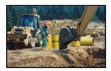
costs. In some cases, site containment is the selected remedy and Shield will execute a design that will include the appropriate type of cap or cover, e.g. RCRA, modified RCRA, asphalt, etc.
